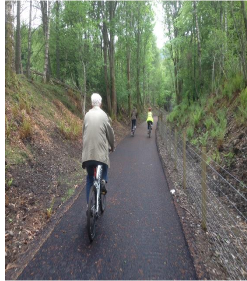
The path uses the trackbed of a disused railway line and has been a popular informal walking route. The path provides 13km of shared surface linking St Fillans to Lochearnhead
